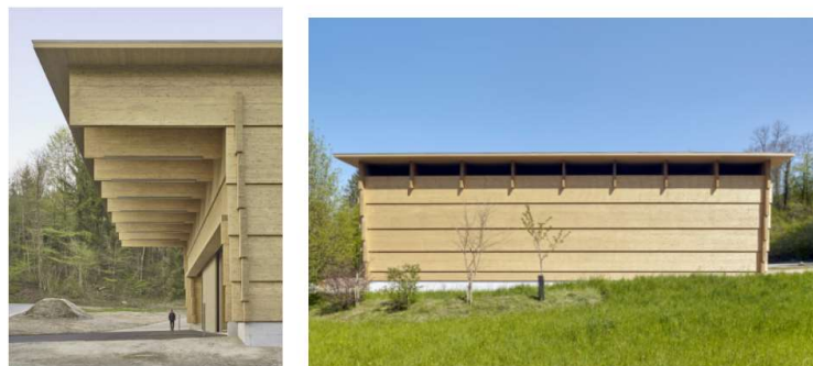
Figure 1 Stacked engineered timber system (Rossetti+Wyss Architekten, 2015)
