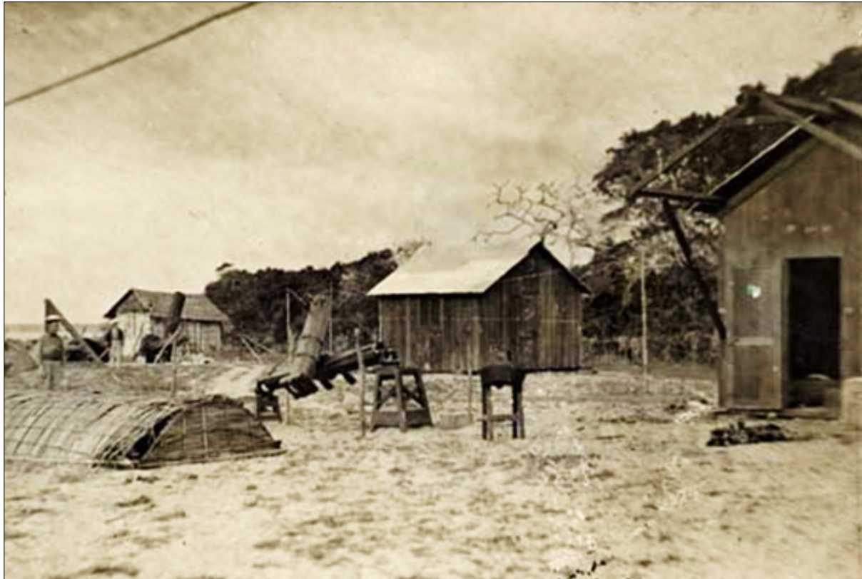
Figure 14: Photograph by Rayet of the French eclipse camp, showing instrument huts and the 40-cm (left) and 20-cm (right) reflecting telescopes set up outdoors (courtesy: Archives, Observatoire de Marseille, 132 J 84).
