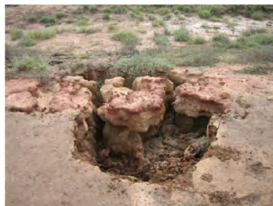
Figure 1 – A typical sinkhole on the levee crest
