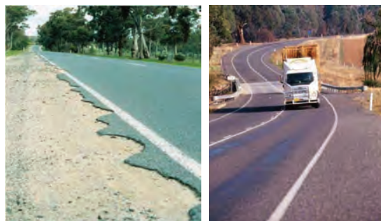
Figure 1 (left) – An unsealed road shoulder with edge deterioration and drop-off; Figure 2 (right) – A road shoulder that has been sealed full width. (Road Safety Toolkit 2010)
