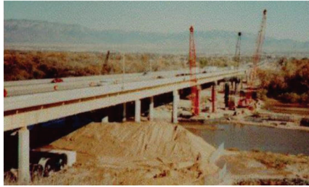
FIGURE 8: I-40 bridge in Albuquerque, USA [41].
