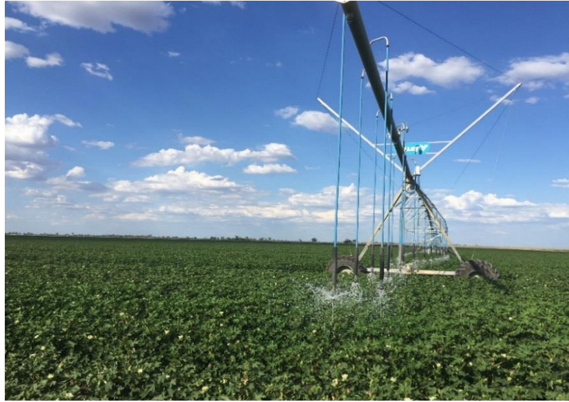
Figure 2.3: Overhead sprinkler irrigation system at Goondiwindi.
