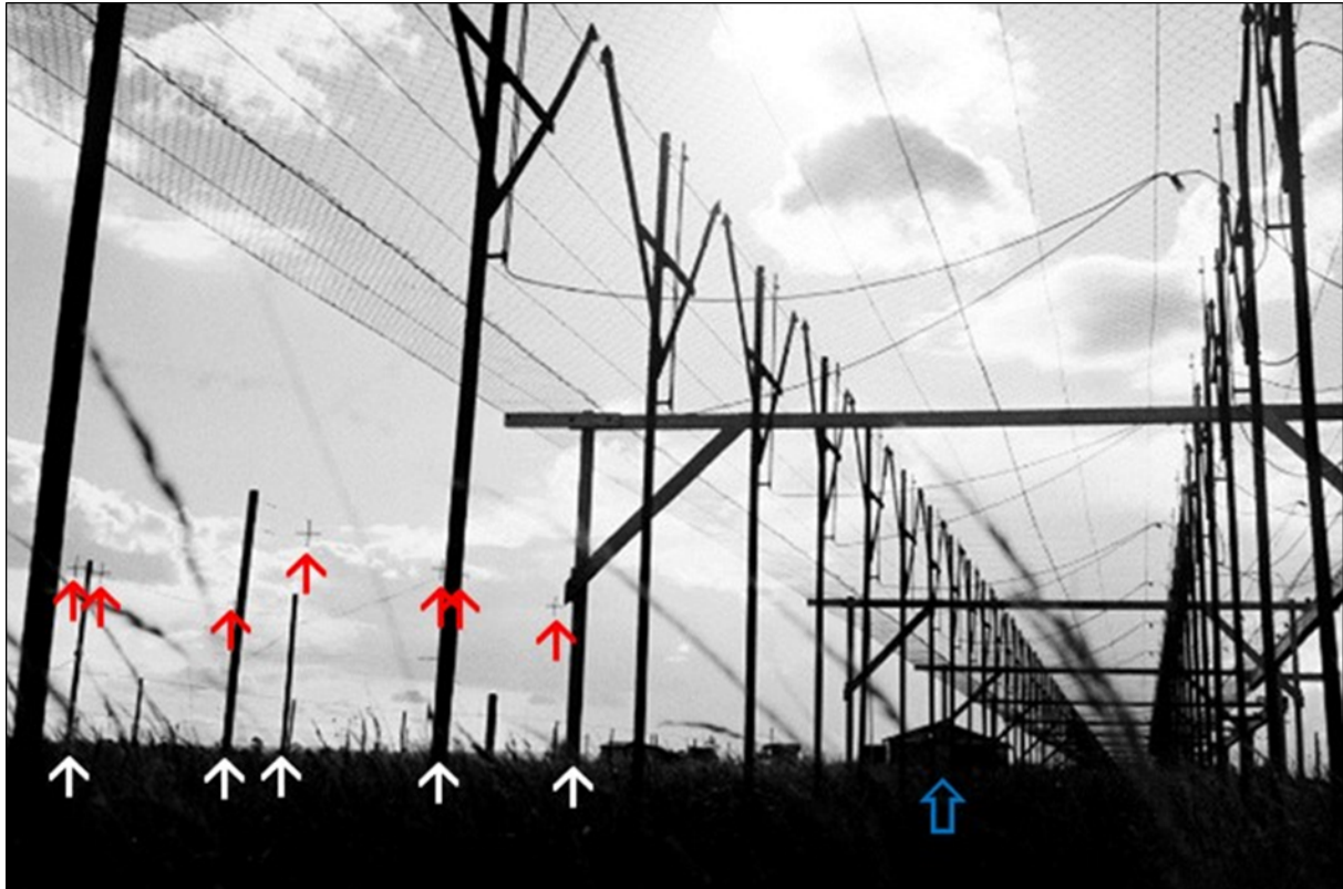
Figure 10: An enlargement of a photograph taken on 30 November 1955 from directly underneath the eastern arm of the Mills Cross, looking west towards the Mills Cross receiver hut (indicated by the blue arrow). On the left (i.e. to the south of the eastern arm of the Mills Cross, are some of the poles (white arrows) that supported the half-wave dipoles of the 14 MHz or the 19.6 MHz arrays. Both radio telescopes had been constructed and were operational by the time this photograph was taken. The second, fourth and fifth white arrows from the left indicate the positions of the poles that supported the first dipole in the array, with the last two poles hidden behind the infrastructure of the Mills Cross. The first and third white arrows mark two of the three poles that supported the second dipole. The red arrows indicate the insulators associated with the first and second dipoles (courtesy: CRAIA, B3868-2).
