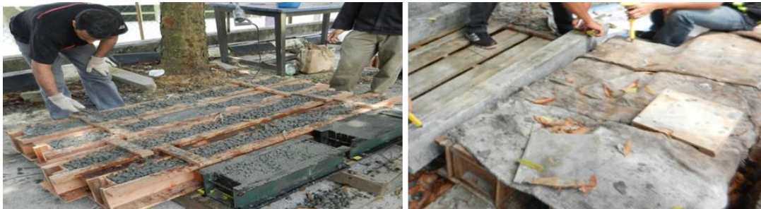
Fig. 3. Casting and curing of RC beams
