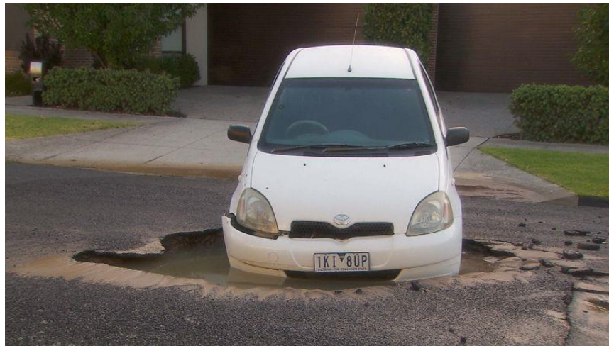
Figure 2.8. A car has plunged into a sinkhole in Gardenvale (9 News, 2019)
