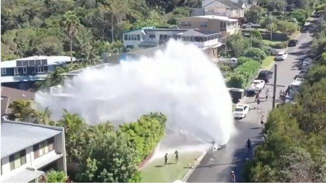
Figure 1.2. A pipe burst in Sydney, Australia (NewsComAu, 2021)
