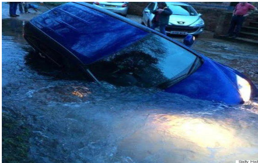
Figure 2.29. Sinkhole 'sucked' car (HuffPost UK, 2016)
