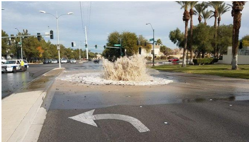
Figure 2.22. Water main break has forced to close the road (Seeman, 2018)
