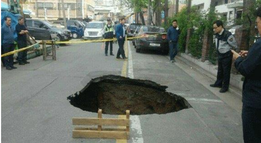
Figure1.1. A sinkhole that opened in Sindorim-dong, Seoul (Herald, 2016)
