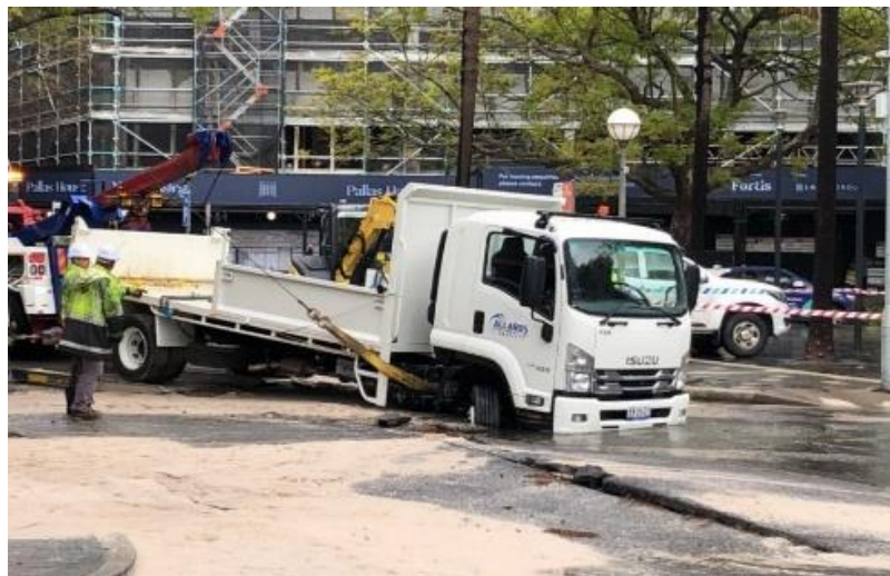
Figure 2.5. A truck got stuck in a road sinkhole (ABC News, 2020)
