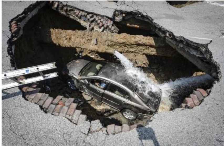
Figure 2.30. Sinkhole has swallowed the car in Toledo (Taylor,2013)
