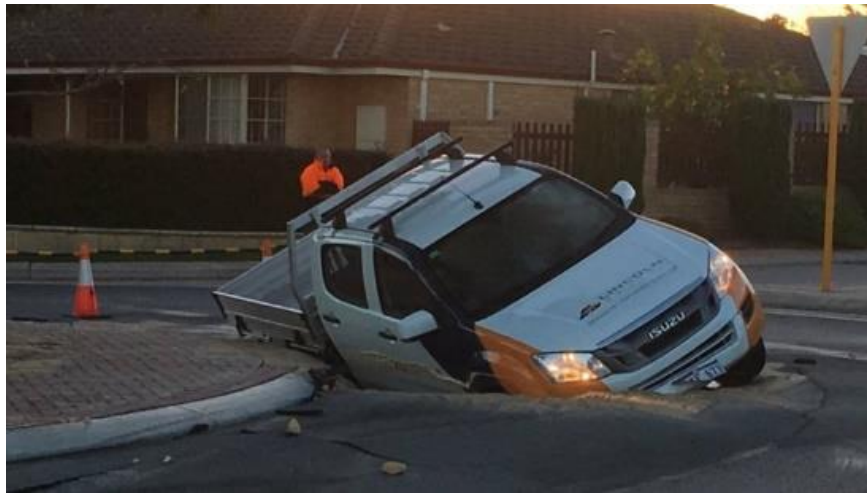
Figure 2.10. Ute was swallowed in sinkhole (Foster, 2017)
