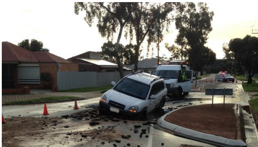
Figure 2.9. A car became stranded in a sinkhole (NT News, 2017)
