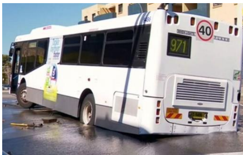
Figure 2.7. Bus stuck in sinkholes due to water main burst (9News, 2019)
