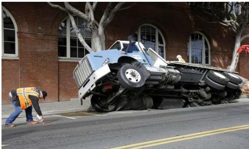
Figure 2.35. The parked truck swallowed into sinkhole (Press, 2017)
