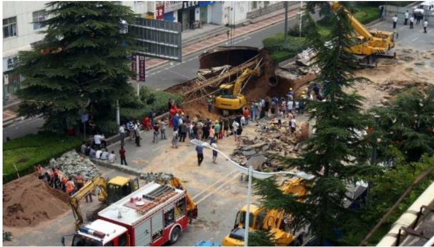
Figure 2.28. Sinkhole opened on a street in China (ABC News, 2016)
