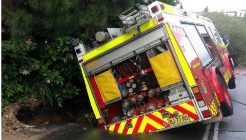
Figure 2.18. Corroded water main burst caused a sinkhole (Sutton, 2014)
