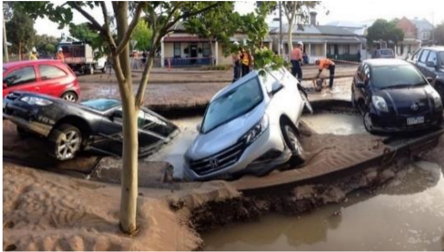
Figure 2.16. Sinkhole opened due to water main burst (ABC News, 2014)
