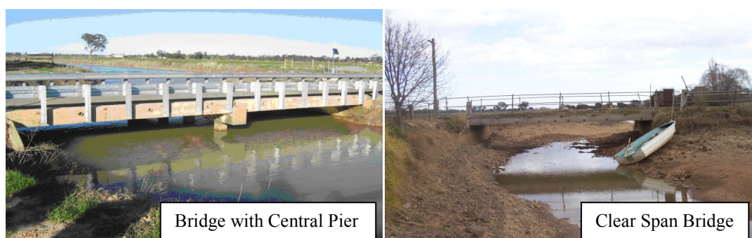
Figure 2.11 Clear span bridges
