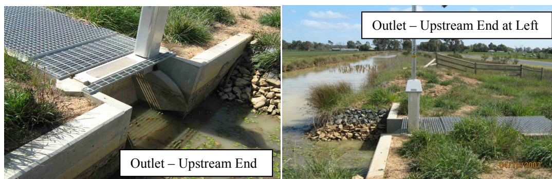
Figure 2.18 Overshot irrigation outlet
