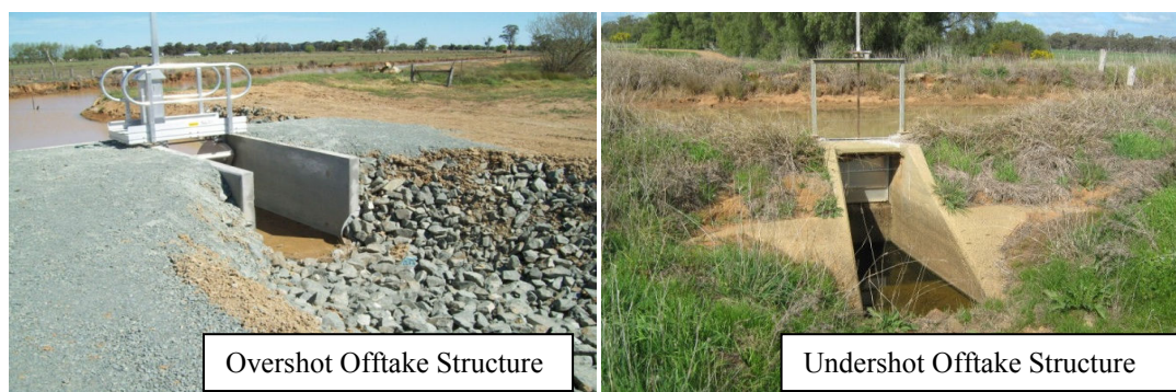
Figure 2.13 Offtake structures
