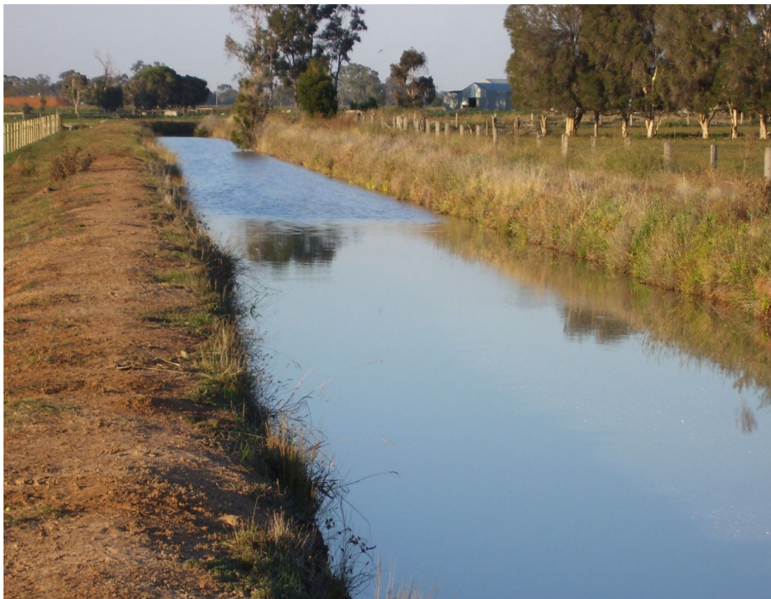
Figure 2.23 Wave damping due to monolayer application (Albrecht, 2011)
