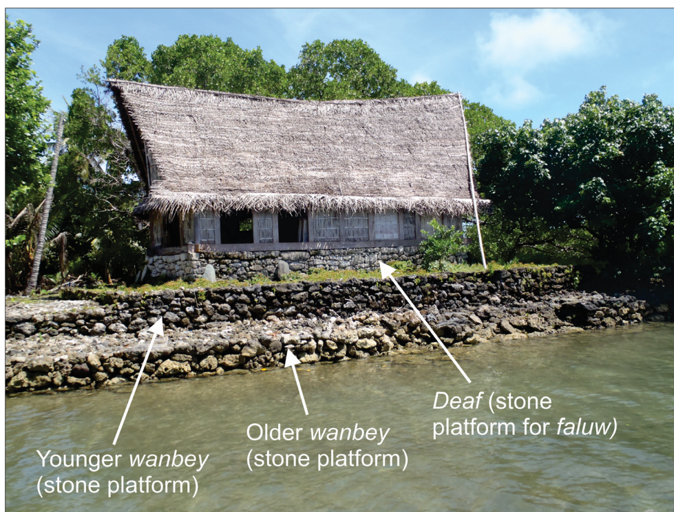
FIGURE 5 The faluw (men's house) at Waalooy, Maap, Yap, showing how an extra stone platform (the younger wanbey ) was added to accommodate rising sea level, a TK-based adaptation to climate change.
