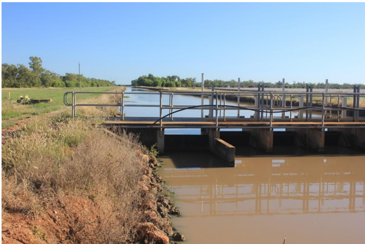
Bundoran Road Channel (Channel B2)
