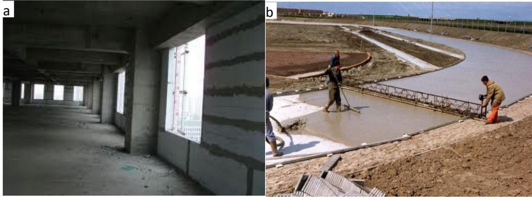
Figure 2. 1 Examples of Foam concrete applications a) insulation wall, b) running track sub-base [36]
