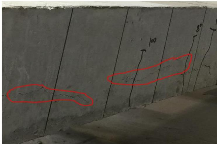
Figure 4. 17 Cracks propagated upward (S3).
