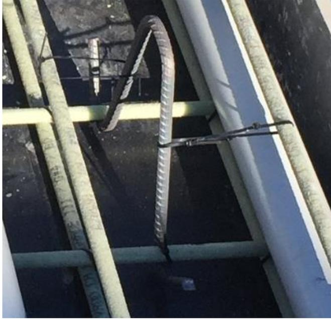
Figure 3.5 Hook used for slab lifting.
