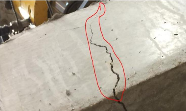
Figure 4.10 Cracks under the point load were wider (S2).
