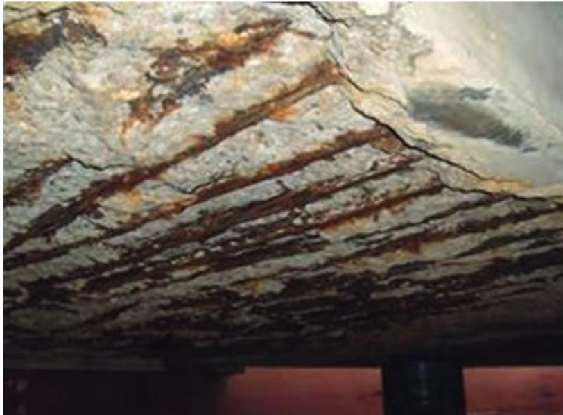
Figure 2.2 Steel corrosion in a structure (Manalo et al., 2014).
