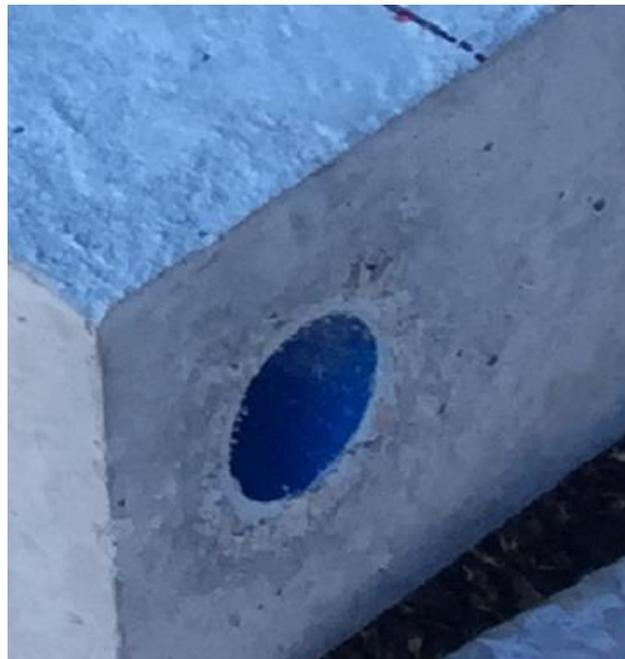
(b) No concrete cracks occurred around the CRS.
