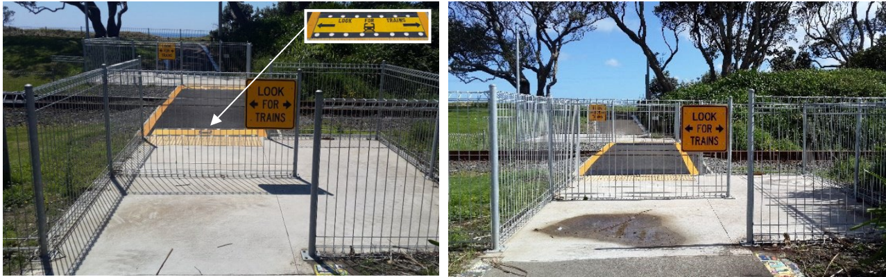
51 Figure 1. View of the level crossing (Left: Trial configuration (with in-ground lights); Right: 52 Standard (control) configuration)
