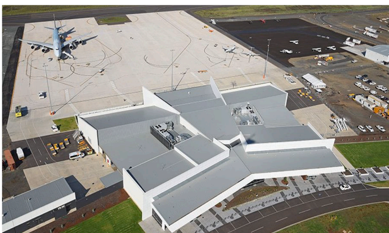
Fig. 14. Brisbane West Wellcamp Airport Australia: World's greenest airport (Supriya et al., 2023).
