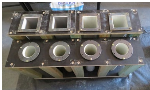
Fig. 3. Formwork of column specimens.
