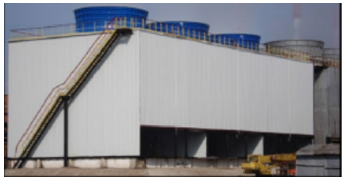
Figure 1.8 Colling tower made from pultruded structural profiles in Russia (Ascione et al. 2016)
