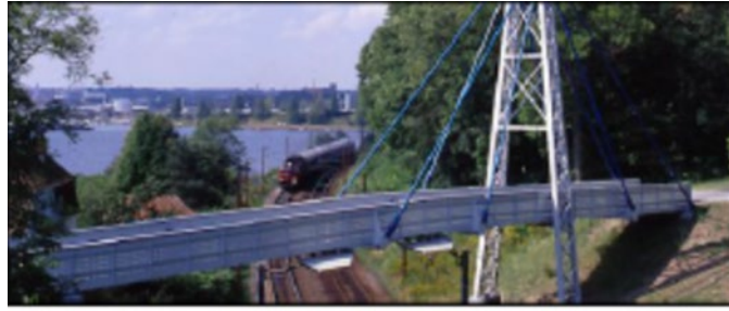
Figure 1.9 All pultruded GFRP Kolding bridge (Ascione et al. 2016)
