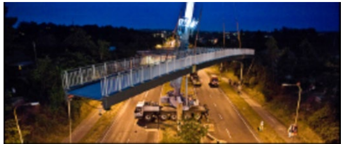
Figure 1.10 Construction of the pultruded FRP bridge (Ascione et al. 2016)
