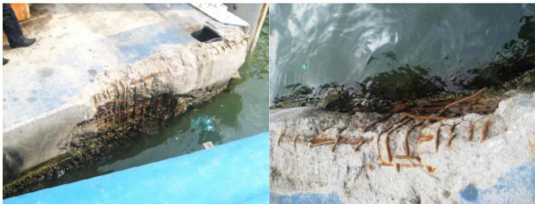
Figure 1.1. Reinforcement corrosion of marine infrastructures (Ramesht & Tavasani 2013)
