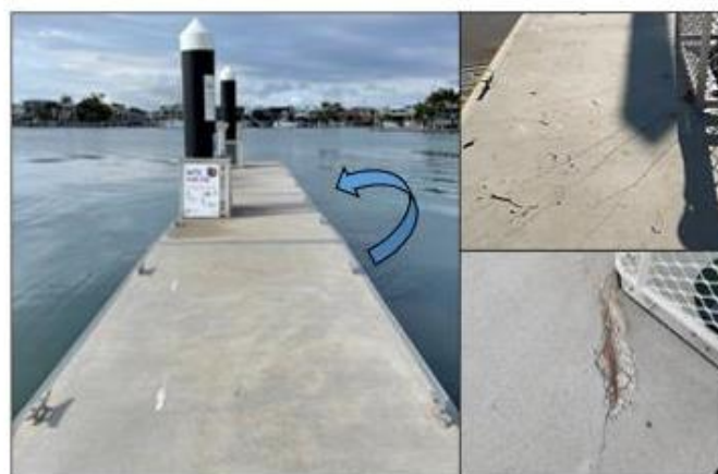
Figure 1. Pontoon in wave action, torsional cracks and reinforcement corrosion.
