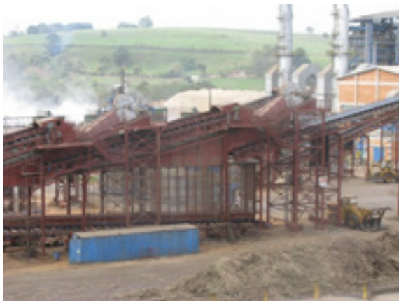
Figure 4.2 Trash recovery from integrated trash and cane delivery in a large sugarmill in Brazil.
