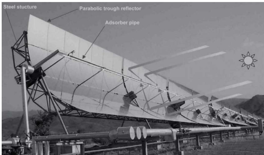
*Figure 2.3: Main components of the PTSC system (Quaschnig & Muriel 2002).*
