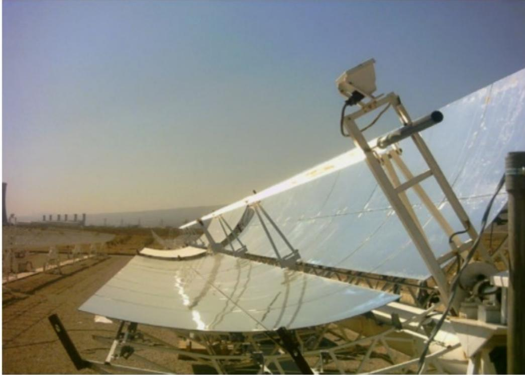
*Figure 2.28: Parabolic collector with absorber tube at Shiraz solar power plant (Naeeni & Yaghoubi 2007).*
