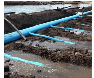
FIGURE 2. Automated system in operation.
