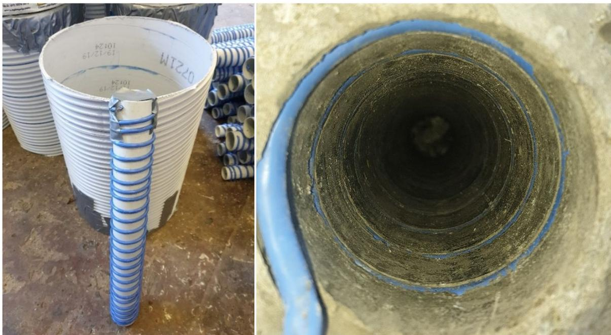
Figure 4 Creating internal rifling on the borehole wall
