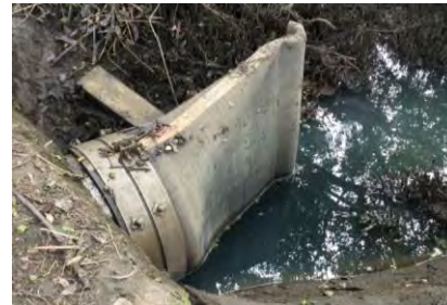
Figure 1: Tideflex “duckbill” valve install installed on overflow relief structure outlet pipe in Norman Creek
