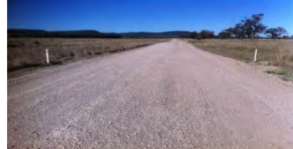
Figure 1 – Unsealed Pavement Example
