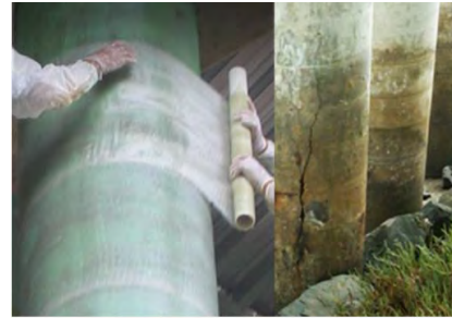
Figure 1 – Rehabilitation using Grout, Resin and FRP wrapping
