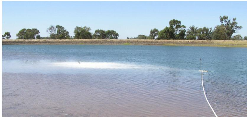
Figure A.22: WaterSavr powder being pneumatically spread from just below the water surface (Brink & Symes 2010)
