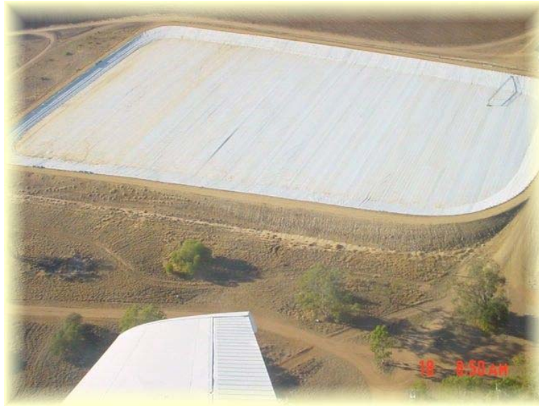
Figure 2 Plastic cover (E-VapCap®) newly installed at Moons Farm, St. George
