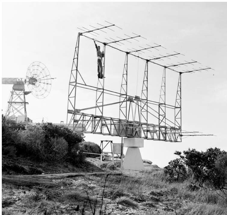
Figure 6.12. Bolton working on the 12-Yagi array at Dover Heights: (above) the view to the south and (below) the view to the north. This array began as an eight-Yagi array in 1951 and in early 1952 was up-graded using cannibalised elements of the earlier nine-Yagi array erected on the roof of the blockhouse (see Figure 5.7). The 12-Yagi antenna was used to carry out the last major source survey at Dover Heights, cataloguing a total of 104 discrete sources. [courtesy: RAIA]
