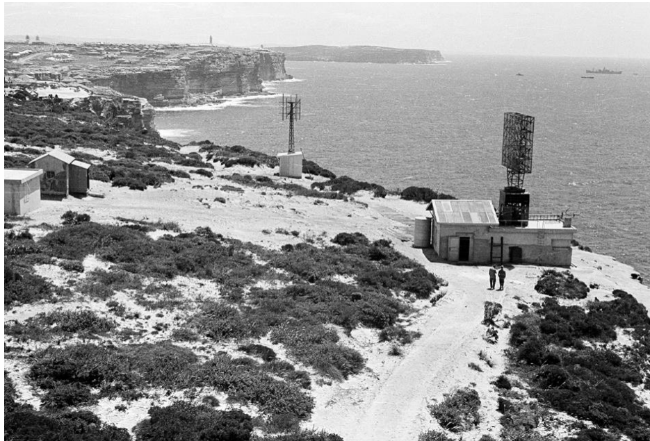
Figure 2.5. The Dover Heights field station operated by the Radiophysics Lab, south of the entrance to Sydney Harbour, in 1943. The radar unit on top of the blockhouse was originally used for the detection of ships along the Australian coast, but then a new version was hurriedly developed for air warning following the Japanese attack on Pearl Harbor in December 1941. The radar unit was removed early in 1947. The cottage at left was occupied by the site caretaker. This site was later to become one of the main Radiophysics field stations for radio astronomy. The blockhouse was to be Bolton's workplace over the period 1946–53. [courtesy: RAlA]
