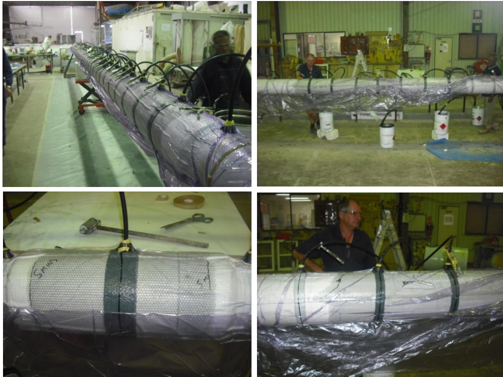
Figure 3.2: Manufacture process of the pile (Courtesy of BAC Technologies Pty Ltd)
