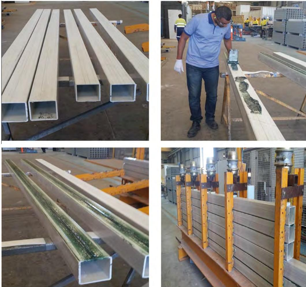
Fig. 1. Preparation process of pultruded sections assembly.
