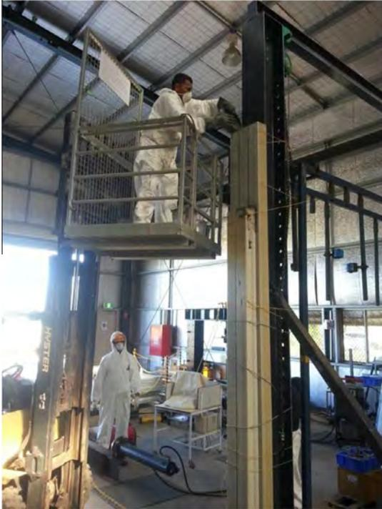
**Fig. 2.** Filling process of the pultruded beams with concrete. (a) Plastic inserts, (b) Steel angles and steel chains.
