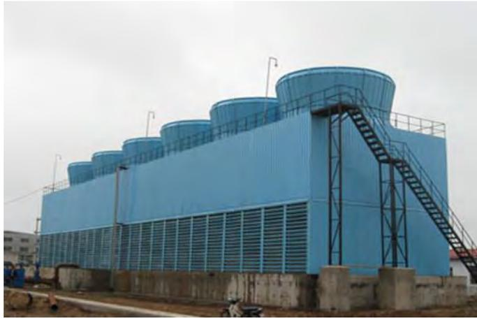
Figure 2.2 FRP cooling tower (Bank 2006a)
