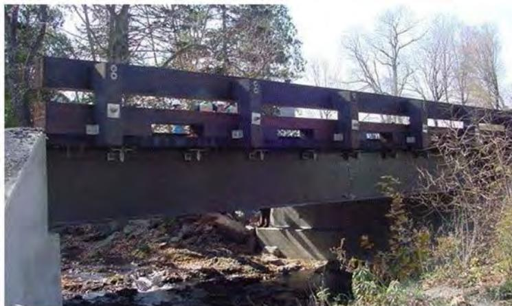
Figure 2.7 FRP DWB girders on Dickey Creek Bridge (Hayes & Lesko 2007)
