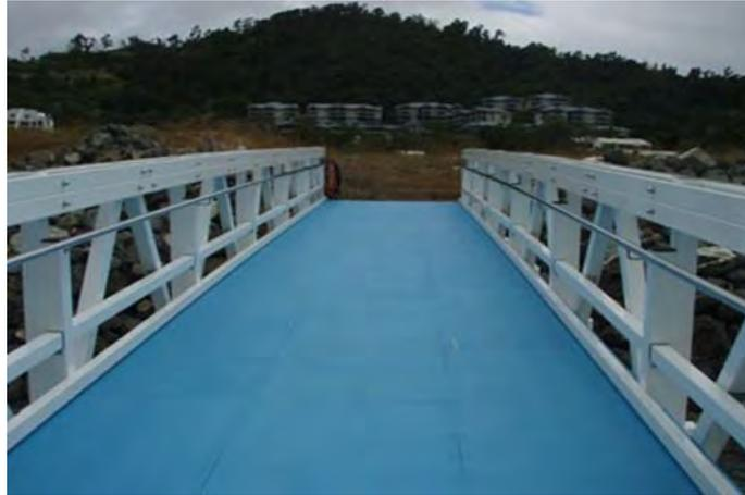
Figure 2.5 Boardwalk bridge using pultruded FRP tubes by Wagners Composite Technologies Ltd, Australia (<http://www.compositesworld.com>)
