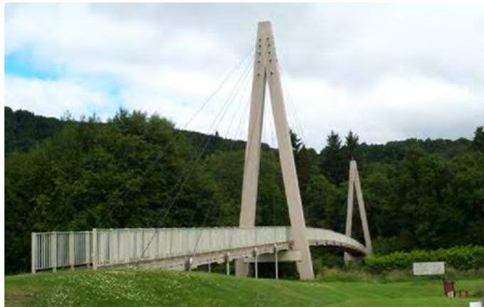
Figure 2.4 Composite decking section footbridge in Aberfeldy, Scotland. (Stratford 2012)
