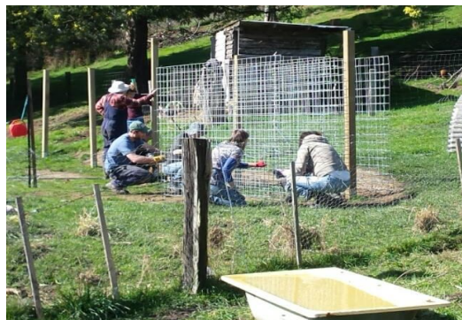
Building the gabion wall: P. Jones
