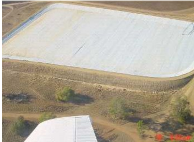
Figure 8 - Plastic cover (E-VapCap®) newly installed near St. George, Qld
