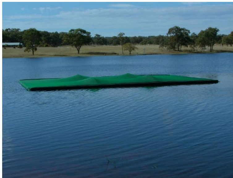
Figure 6 - Shade cloth installed as a series of floating modules to avoid suspension cables
