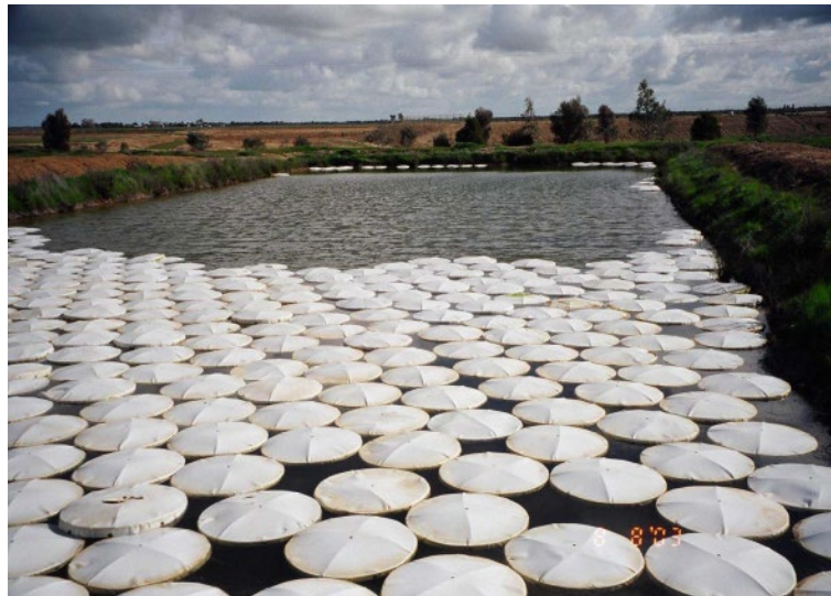
Figure 11 - AquaCaps - a prototype circular design of modular cover
