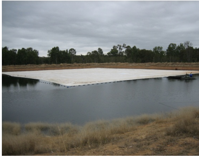
Figure 9 - Deployment of floating cover (E-VapCap®) as a floating raft
