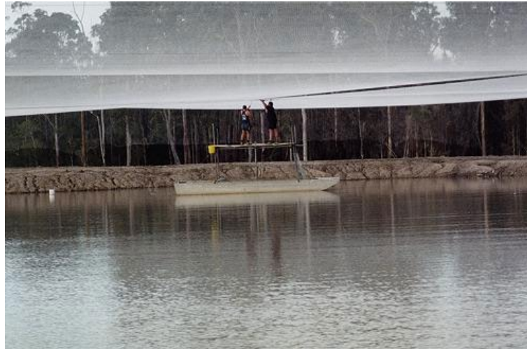
Figure 5 - Installation of suspended shade cloth cover
