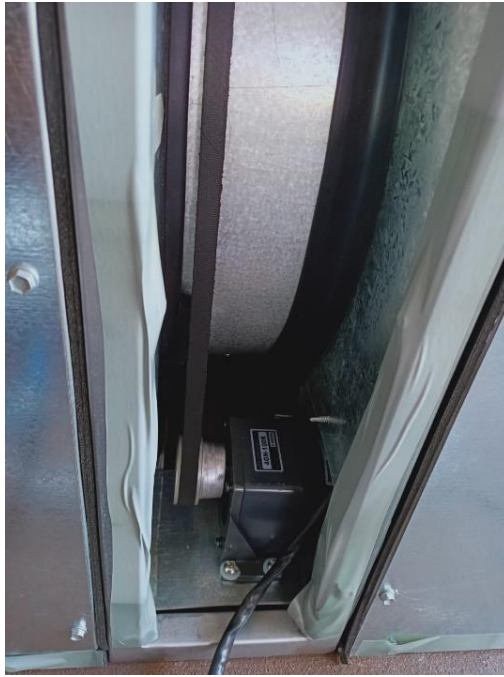
Figure 4.5: The DW driving system including the motor attached with a gearbox and pulley connected with the DW by A-section industrial V belt, which located at the bottom left corner in figure 4.4.
