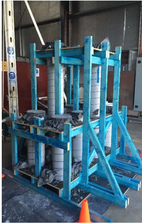
Fig. 6. Wooden framework and plastic formworks with cast column specimens.
