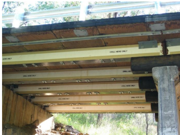
Fig. 11. FRP sandwich bridge beams (Van Erp and McKay, 2012).
