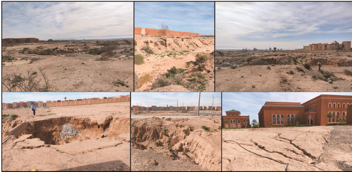
Fig. 12. Photos showing the influence of gully erosion on the infrastructure within the study area.
