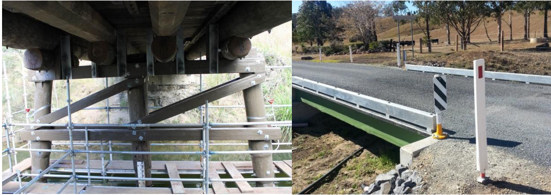
Figure 2-2: FRP Highway Bridge Structures: a) Components for Timber replacement (2013) and b) Monolith Highway Bridge Deck (2014)
