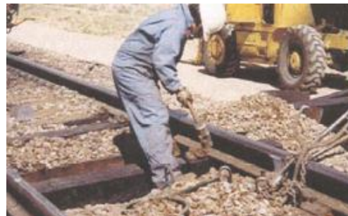
(b) Installation of recycled plastic composite ties
