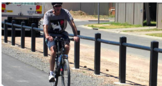
(a) Fencing in South Australia
