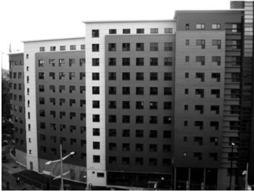
Figure 2.28: Modular twelve floor student accommodation building in Bristol [152]
