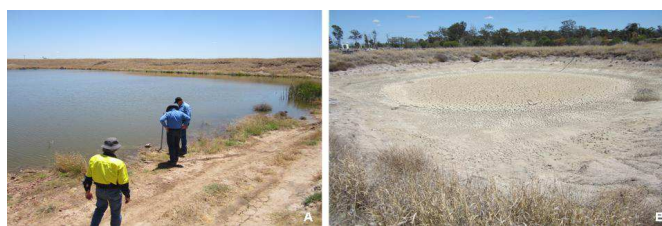
Figure 1. Photographic examples of an operating CSG dam (A) and a dam after evaporation of produced water (B) in the Bowen Basin in central Queensland, 2013.
