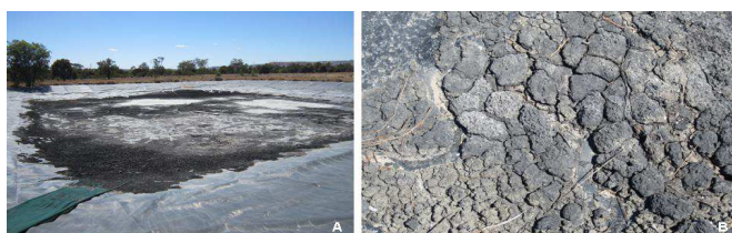
Figure 2. Photographic examples of CSG evaporation dam after dewatering (A) and close up of CSG sediment (B) in the Bowen Basin, 2013.
