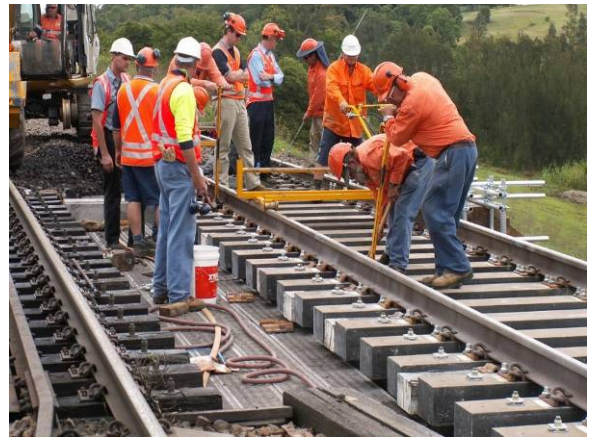
Figure 4. Sleeper made of polymer concrete and fibre composites
