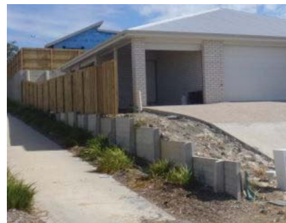
Image 1 – Sample image of retaining wall on property boundary
