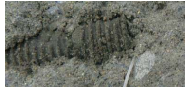
Figure 1 – Protective FBG Sensor Encasing Successfully Bonded to Concrete
