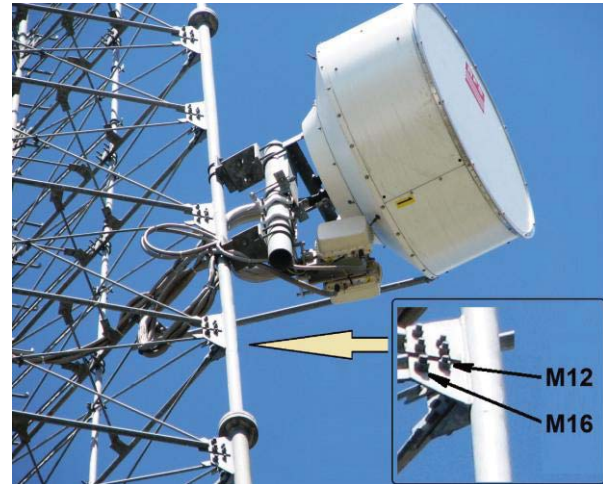
Figure- 1: Typical arrangement of bolts on towers
