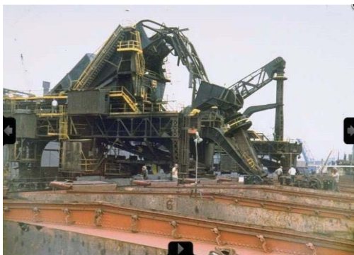
Figure 1: Fatigue Damage of structure ("Leap Australia," 2014)
