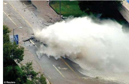
Figure 1 – Burst Water Main (Associated Press, 2014)
