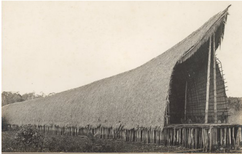
Figure 9. Dubu daima at Kaimare, Urama Island. Note the high density of house post supports (Hurley 1921).
