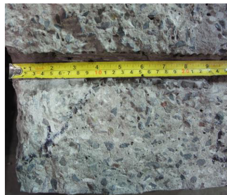
Fig. 8. Zone of concrete deformation due to cable bending in shear.
