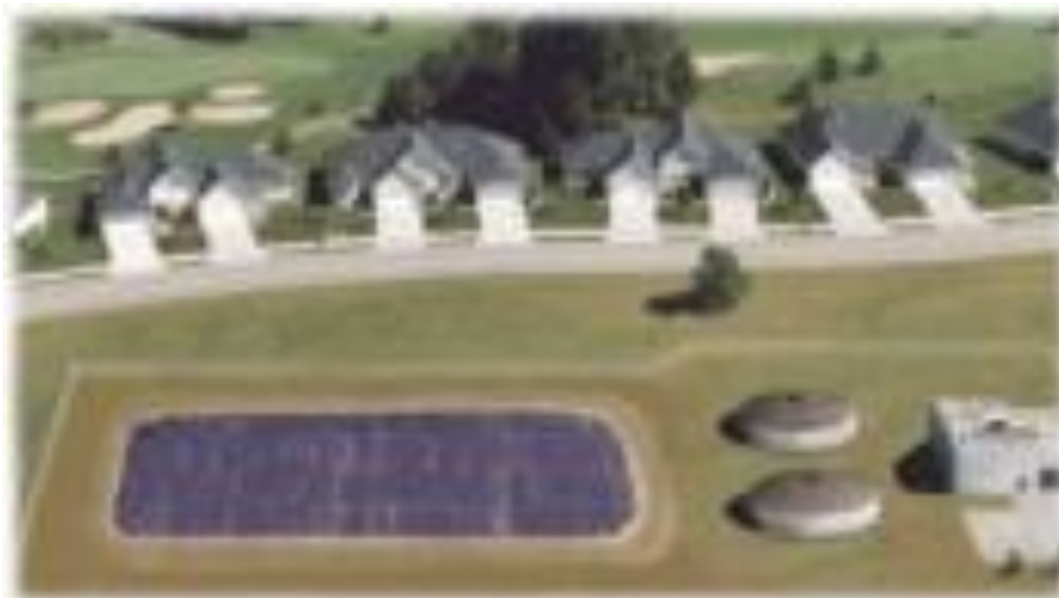
Lagoon of activated sludge
