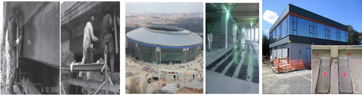
(a) Rehabilitation of a RC superstructure by using CFRP wraps; Muddy Creek Bridge, Preston County, WV (October 2000) [169]
