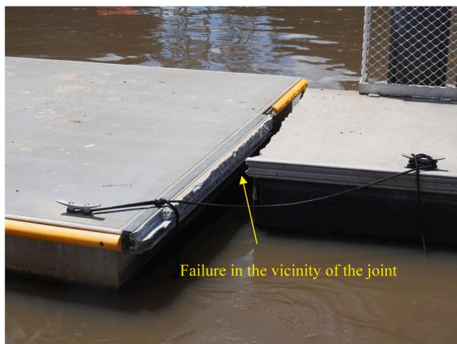
Fig. 1. Localised damage near the joint on the pontoon decks during the 2022 Queensland and New South Wales flood.
