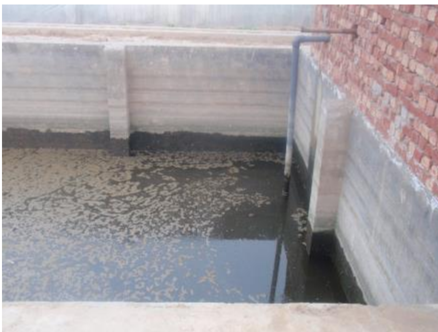
Figure 4.23: Reservoir constructed at the drip system site to store the water.
