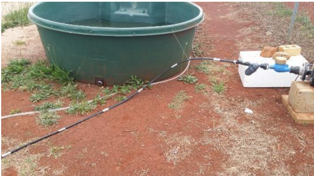
Figure 3.10: Sealed extra dripline connecting water supply to the 100 m dripline.
