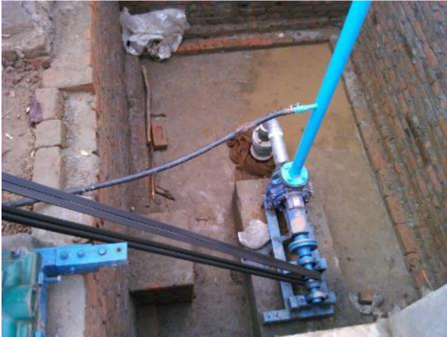
Figure 4.8: Water pump with electric motor installed at the pump shed.
