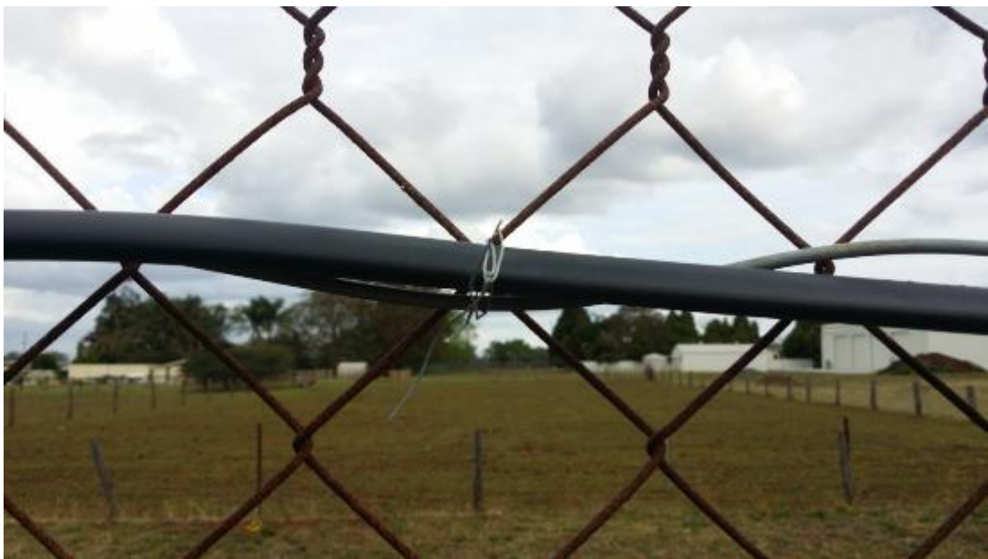
Figure 3.14: Dripline attached to the fence at agriculture plot area using steel tie wires.
