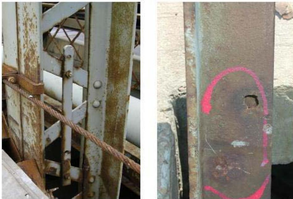
Figure 1.1: Corrosion effects on low level Bridge Northbound (Lima et al., 2008)
