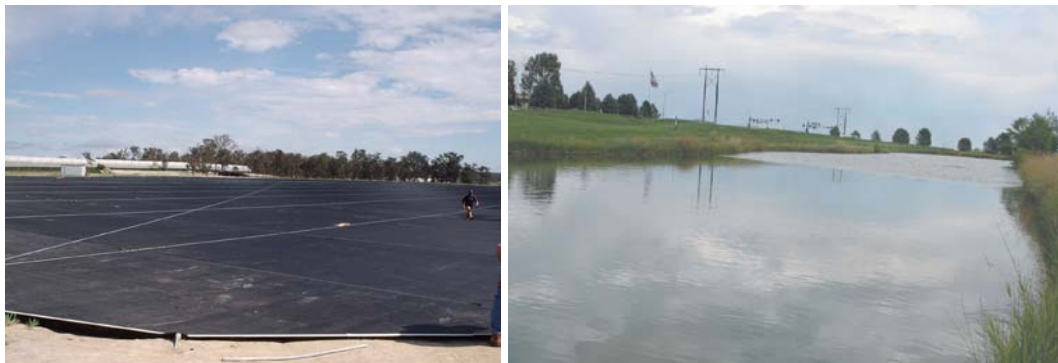
Figure 4: Examples of Evaporation control products: Top left : Continuous floating cover; Top right : Modular System; Bottom left : Shade Cloth Structure; Bottom Right: Chemical Monolayer
