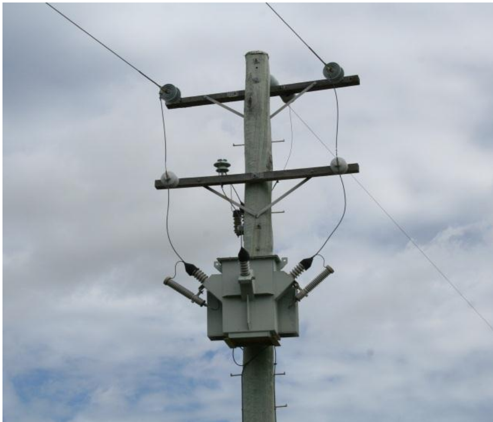
Figure 2.3: SWER line isolating transformer [2].
