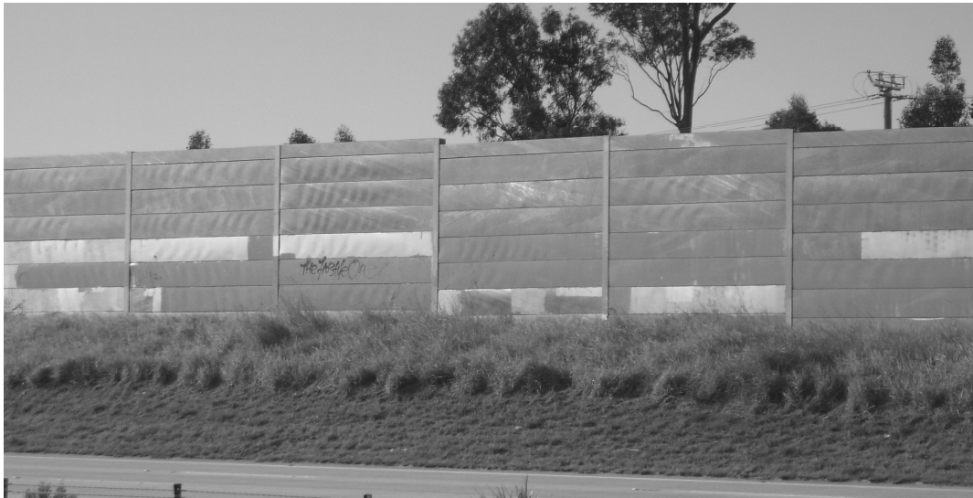
Fig. 4: A section of the NB12 noise barrier along the M1 Motorway.
