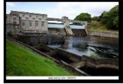
Figure 5.3.6. Pitlochry dam and fish ladder
